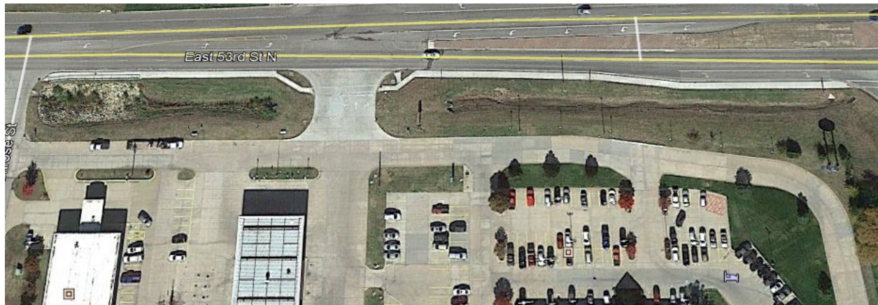
53 rd Street Large Drainage Ditch Google Earth Image
